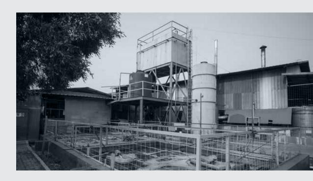
PT. Pelangi Elasindo is an environmental conscious company. Thus, we go to great lengths to build a wastewater treatment facility that includes coagulation, flocculation and biological processes. We reuse the discharged water back into production, recovers heat through heat exchangers and reuse boiler's condensate. We are doing everything we can to protect and preserve our fragile environment.
